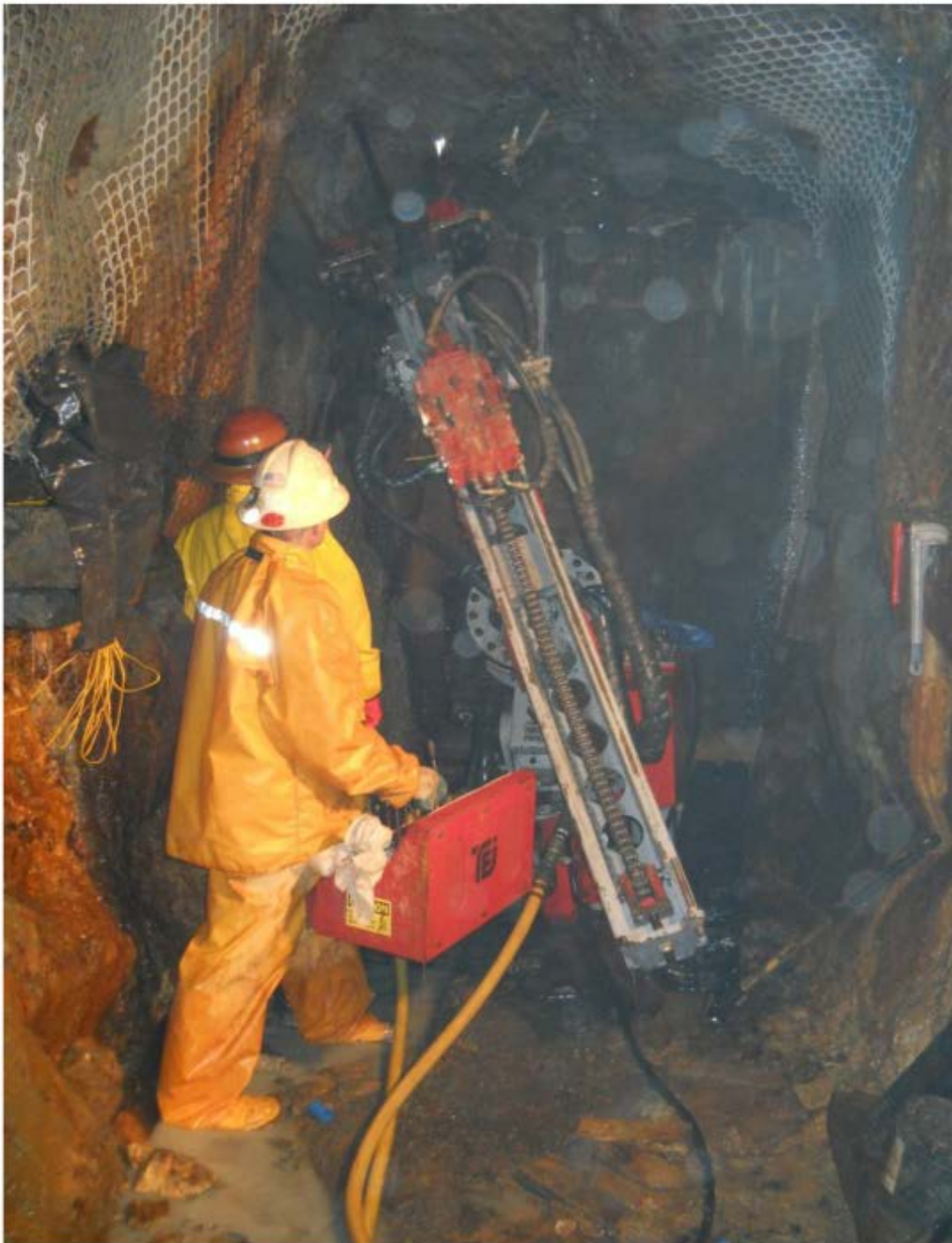
Grouting Koehler Bulkhead
