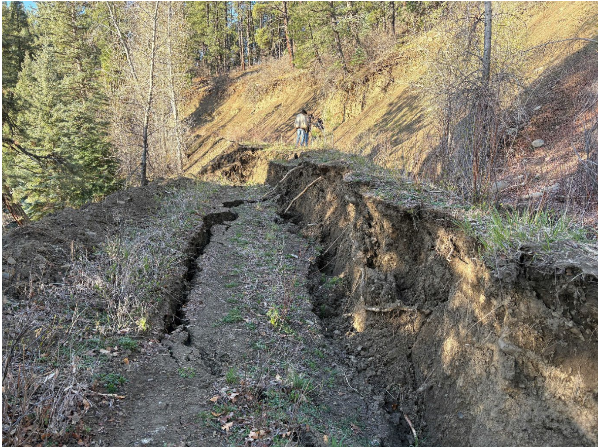
Ditch bank failure looking south
