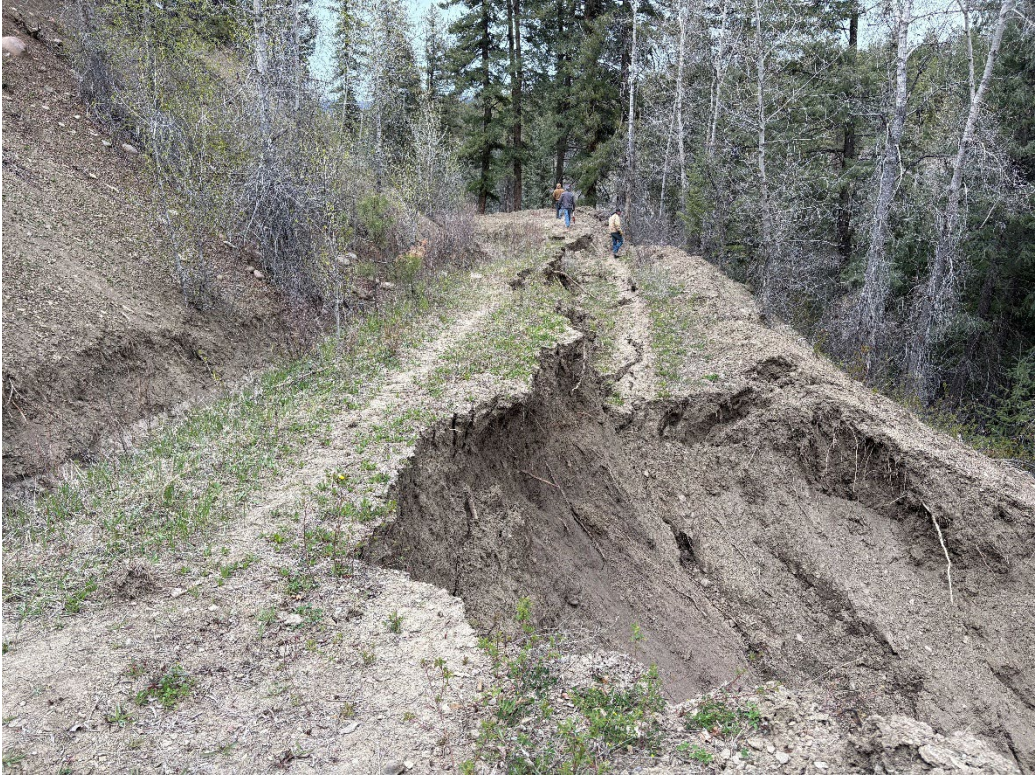
Ditch bank failure looking north
