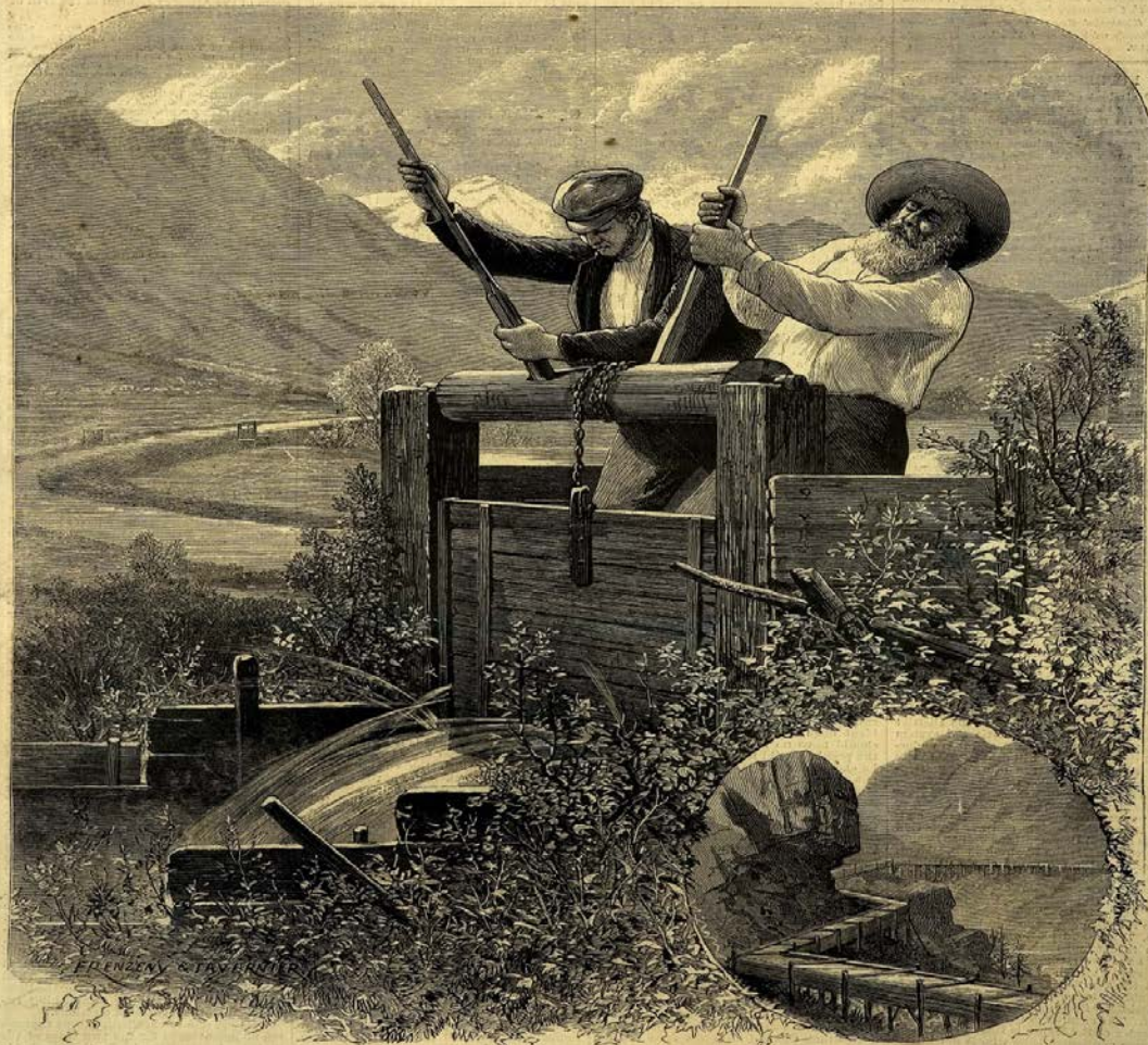
IRRIGATION IN COLORADO—LETTING WATER INTO A SIDE SLUICE-WAY.—[SEE PAGE 514.]
