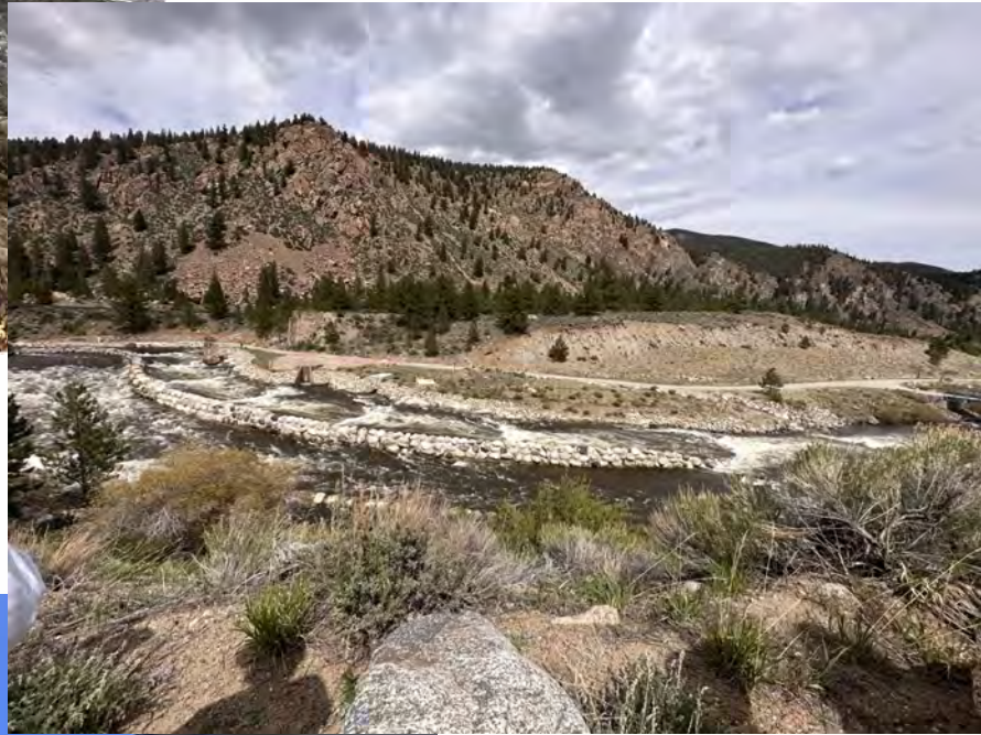
Safe boating passage/fish ladder diversion
