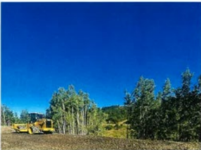
Photo of repairs: October 25, 2023
