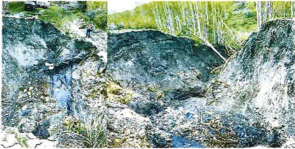
Figure 1. Breach 1 (right) and erosion (top left)
